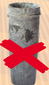
Rapid corrosion of untreated Aluminium
